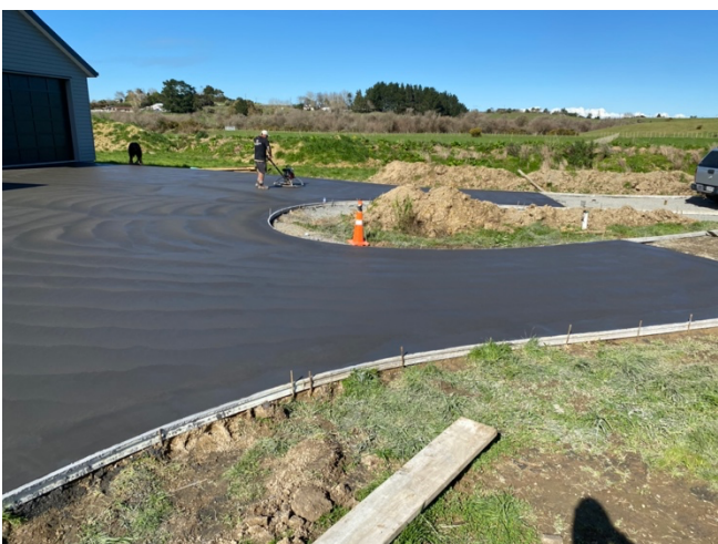
Fresh powerfloat lines, these will fade over time
