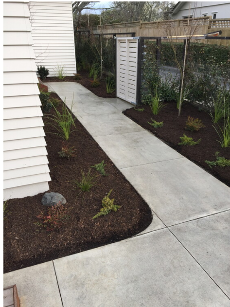
Plain concrete acid etched and sealed (no oxide)
