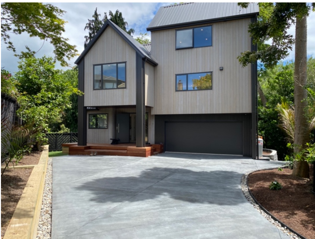
Half charcoal driveway acid etched and sealed
